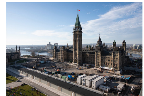
Centre Block Rehabilitation (2021–2031)
