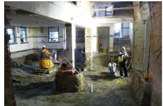
Excavating for Basement Footing 1914 Block Quadra, B.C.
