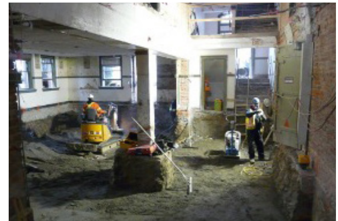
Excavating for Basement Footing 1914 Block Quadra, B.C.
