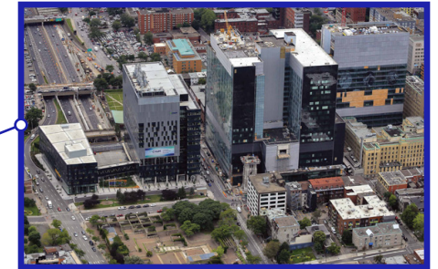
Health District → CHUM hospital complex. © Helico/Construction Sante Montréal.
