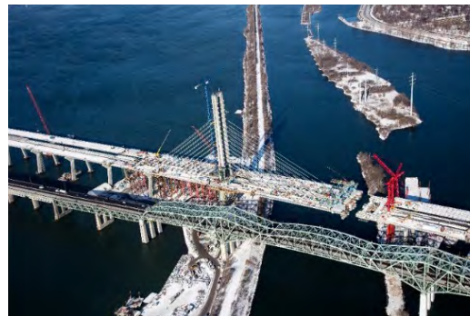
Construction of the asymmetric 240-m cable-stayed main span with 168-m high concrete tower
